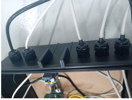
Figure 8: Cable glands installed on the box
