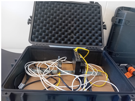
Figure 3: Box before modifications
