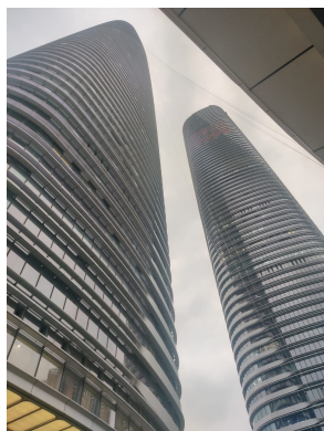
FIGURE 1 – Galaxy Twin towers, Linxai headquarters in Shenzhen, China
